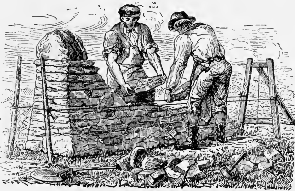
Fig. 364.—Mode of Building Stone Wall.
